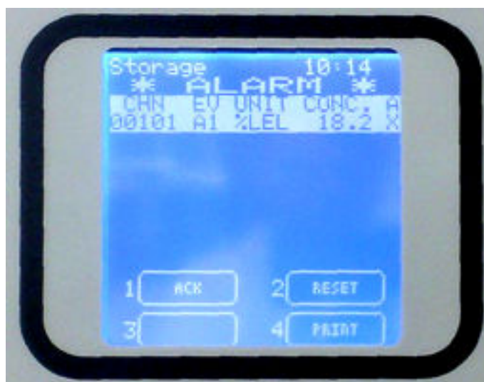
Fig. 3.2.1.b) Typical ALARM state of the ACTIVE EVENTS screen.
