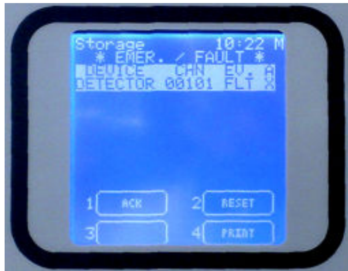
Fig. 3.2.1.d) Typical FAULT state of the ACTIVE EVENTS screen.
