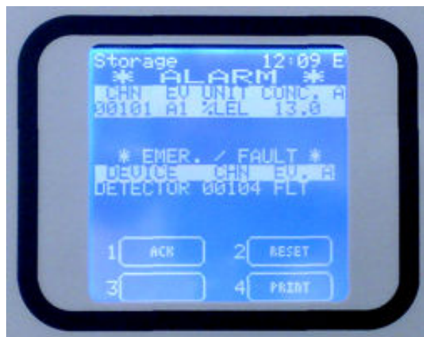
Fig. 3.5.1 a) Active Events screen with Alarm and fault
